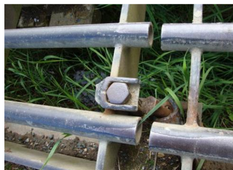
Longitudinal gap greater than 15mm
