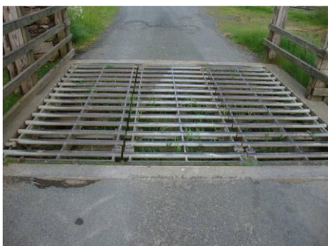
Longitudinal gap greater than 15mm
